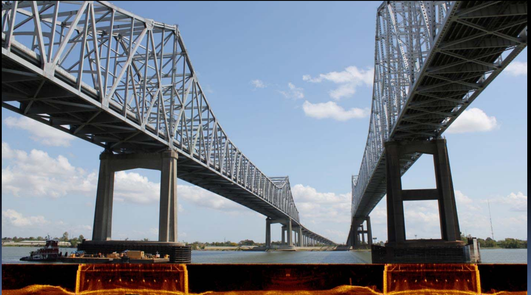
Crescent City Connection, and Greater New Orleans Bridges New Orleans, LA
